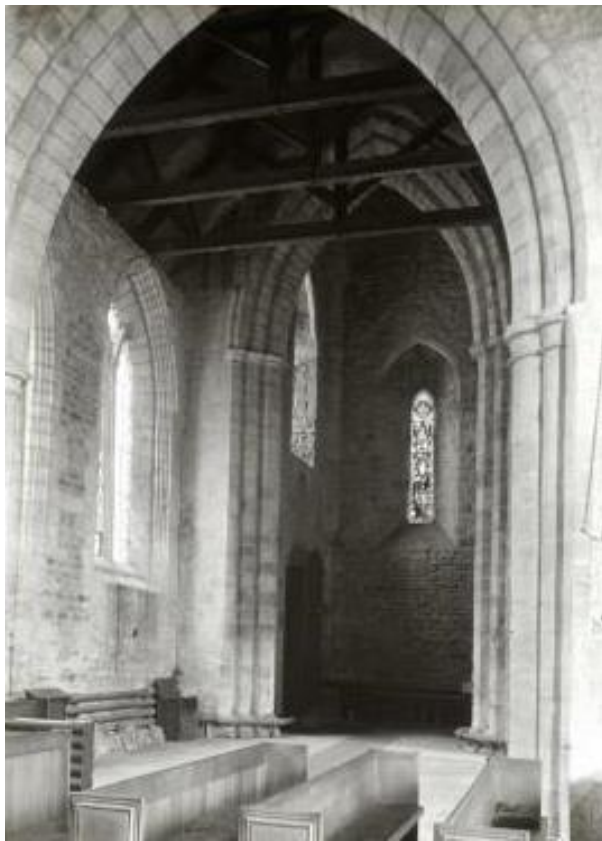
Pl. 9: The North Transept, showing the arrangement of heating pipes associated with the boiler house.
