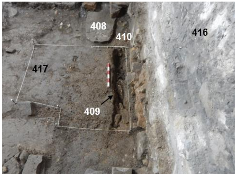
Pl. 4.8: Trench 4 from north showing natural (417) under (408), cut by foundation trench of wall (416) (409) with fill (410).
