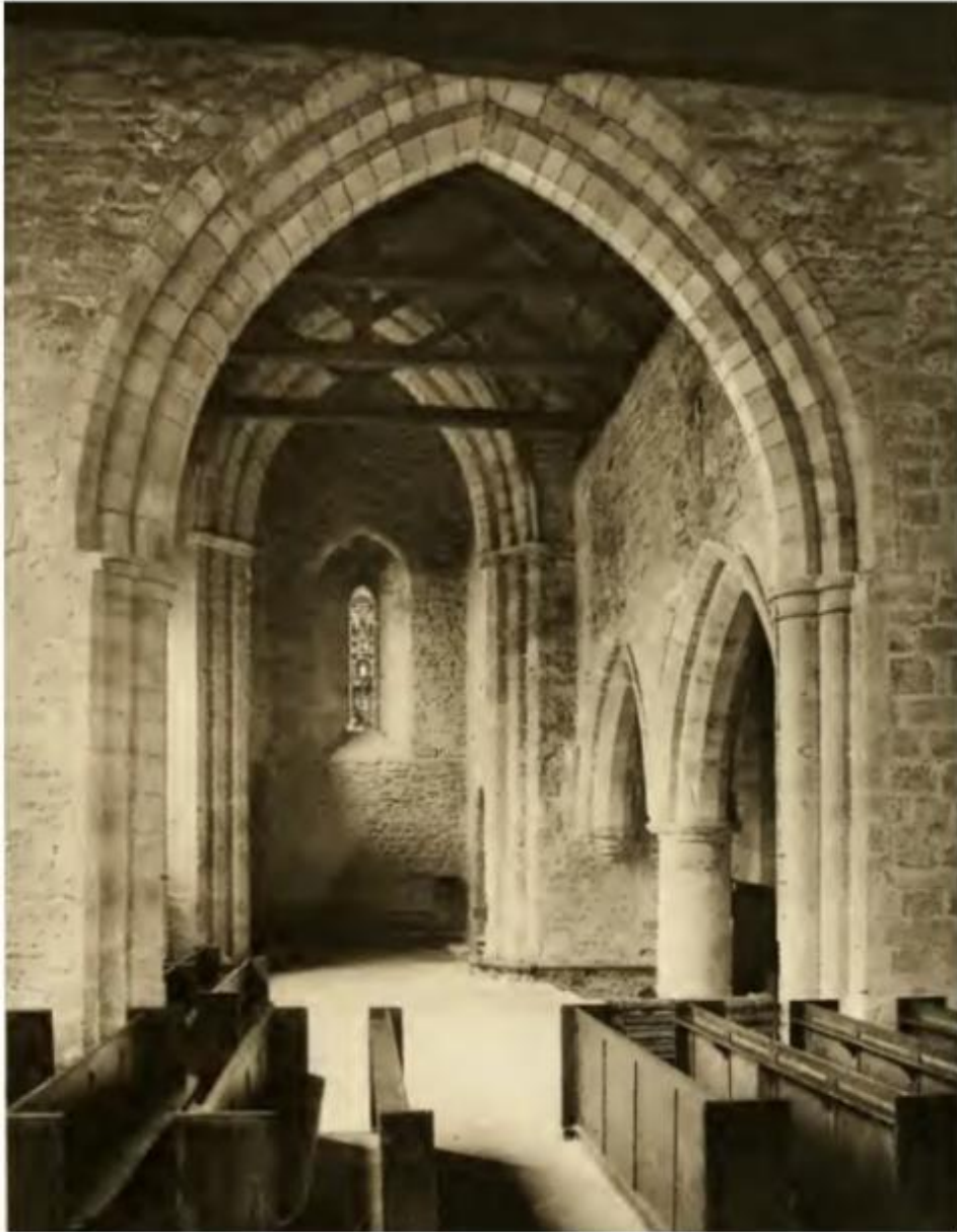
Pl. 7: The exit of the former flue through the wall can be seen on the right, just beyond the arch in the foreground and above the nearer arch of the aisle 67 .
