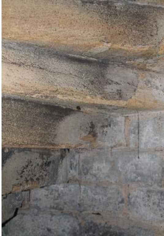
Pl.1: Ashlar stonework and underside of stair treads.
