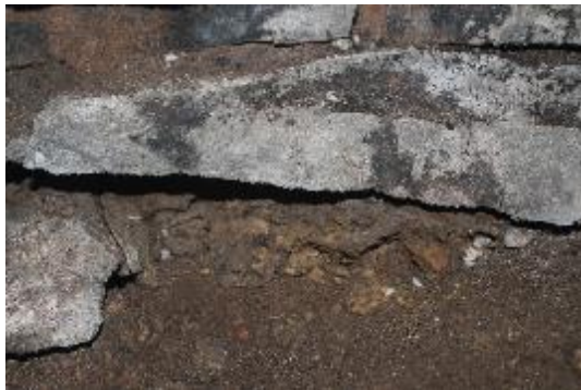
Pl. 4: Foundations of tower on boulder clay.
